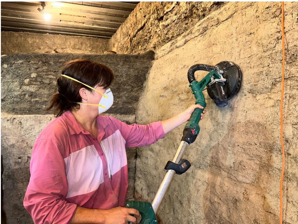
Figure 6. Using floor sender on Profile K to smoothen the render surface
