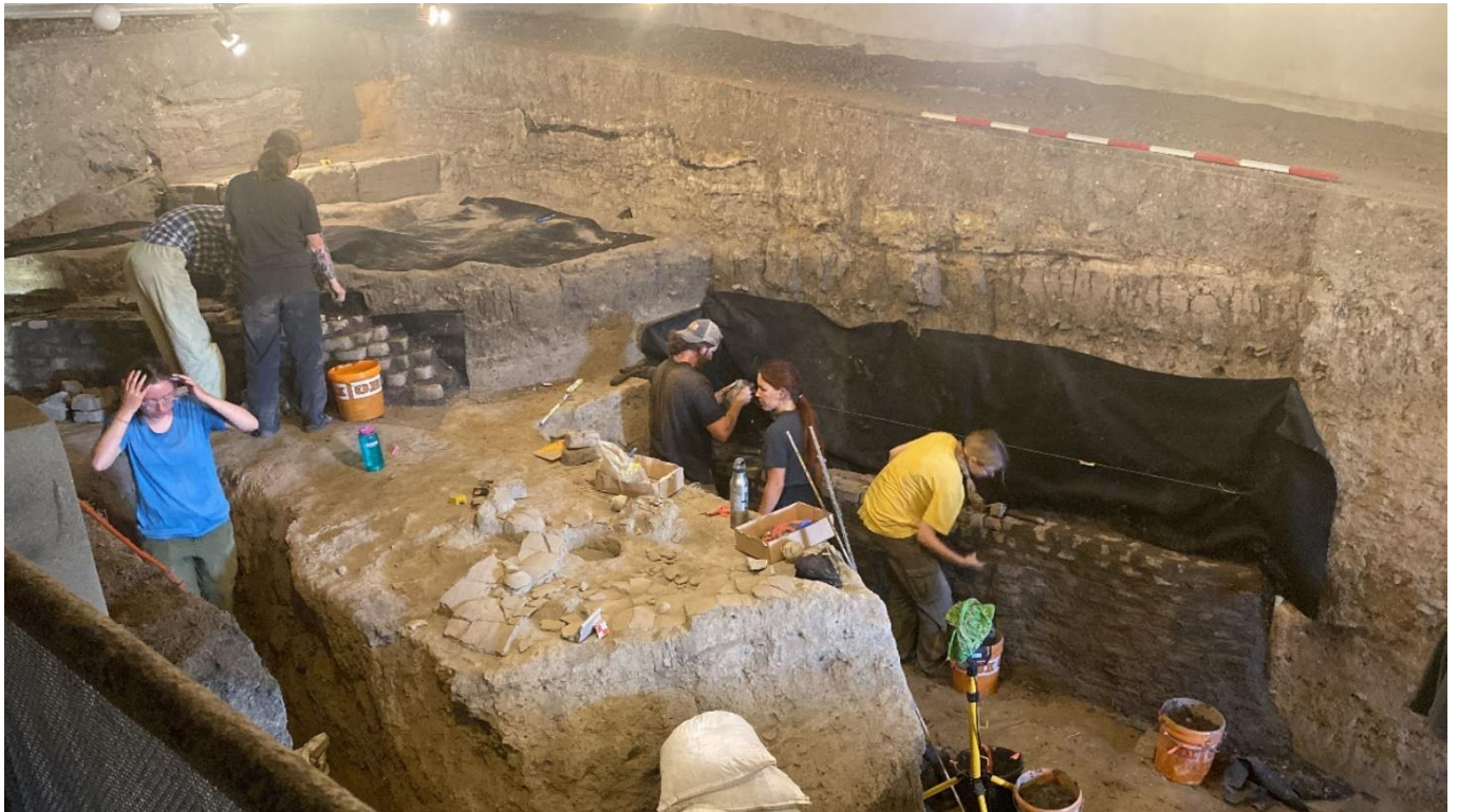
Figure 10. Sacrificial support structures in Profiles F and K, and a protective geotextile layer on Platform E in Season 2023
