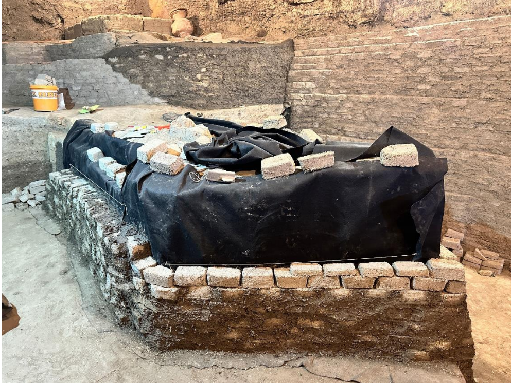
Figure 5. Construction of a sacrificial support structure along Profile H
