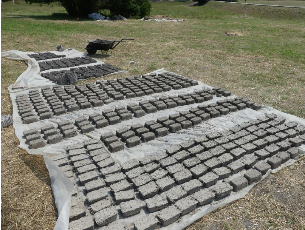
Figure 9. Mudbrick production for sacrificial support structures in Season 2023
