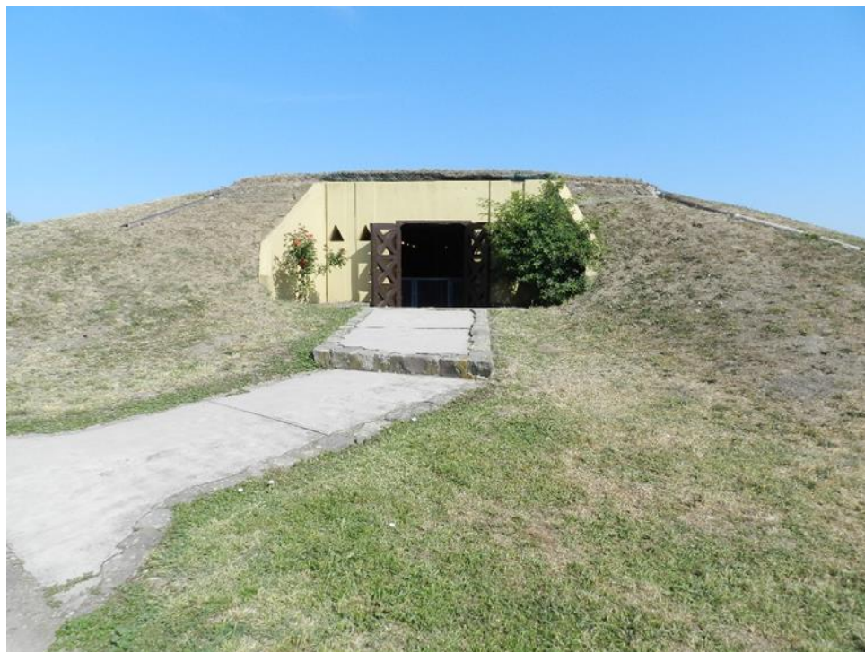
Figure 4. The entrance of the shelter to the in situ exhibition
